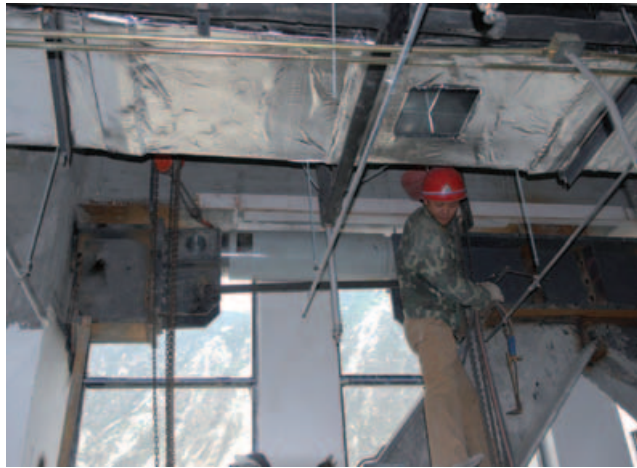
Figure 5. Installation of viscous damper
